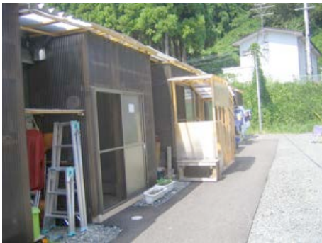
Housing units are built in a row over loose gravel, making access difficult: the wheelchair ramp faces the back of the housing lot, making it difficult for the elderly residents to enter their own home.
